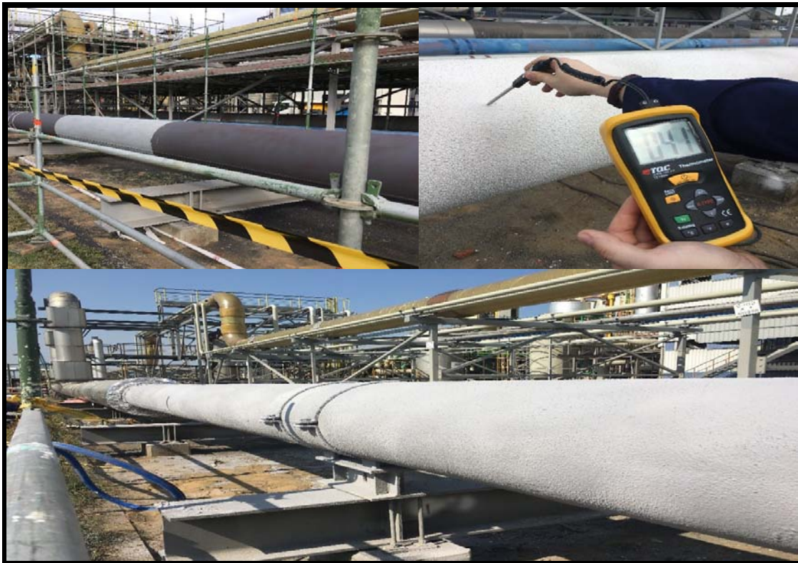
Figure 2: TGPS CUI mitigation system.
